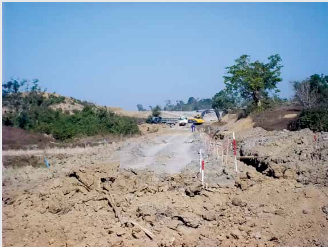
Figure 3 Daewoo clearing pipeline route for the offshore gas terminal, Arakan state. SGM, 2011.
