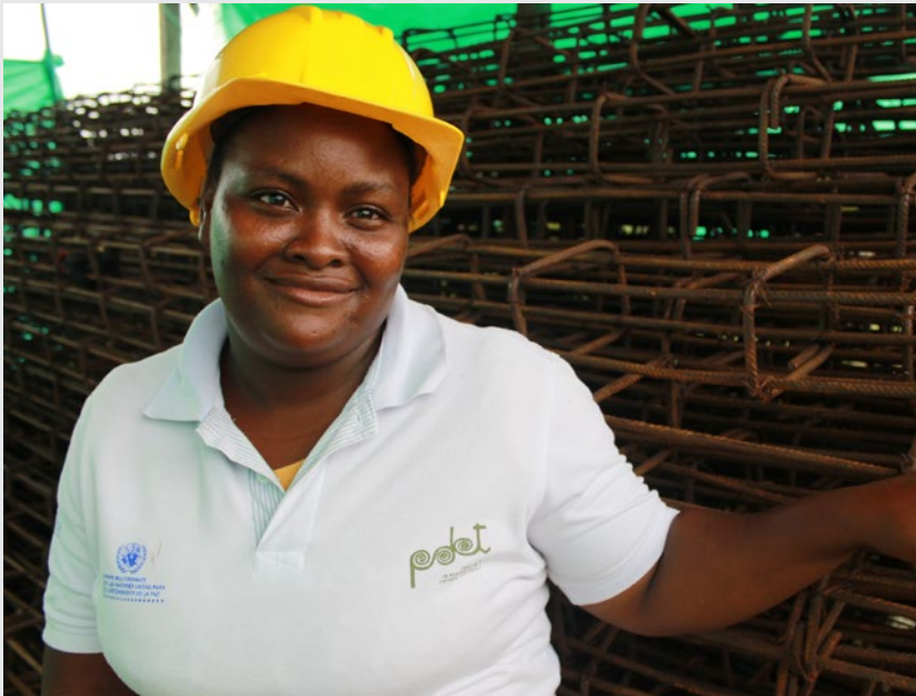
Luz Nery Salon pictured at the road construction site where she works (photo courtesy of UNDP, Colombia).
